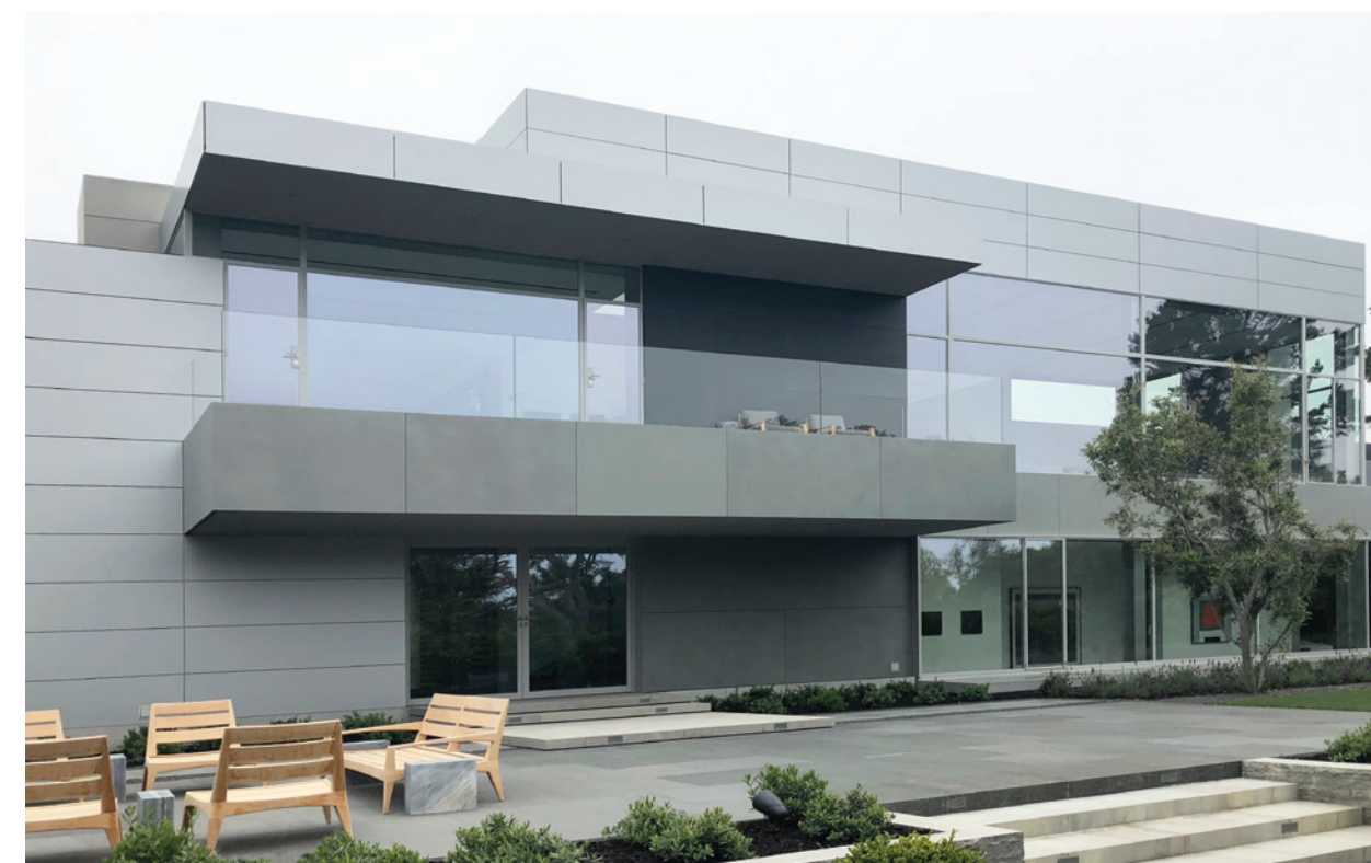
PLANAR PLAY At the back of the house (this photo), poured concrete cross walls define bedroom terraces. At one end is a parking area and the garage (below, left). The entrance vestibule also opens to a large terrace on the east (below, right).
